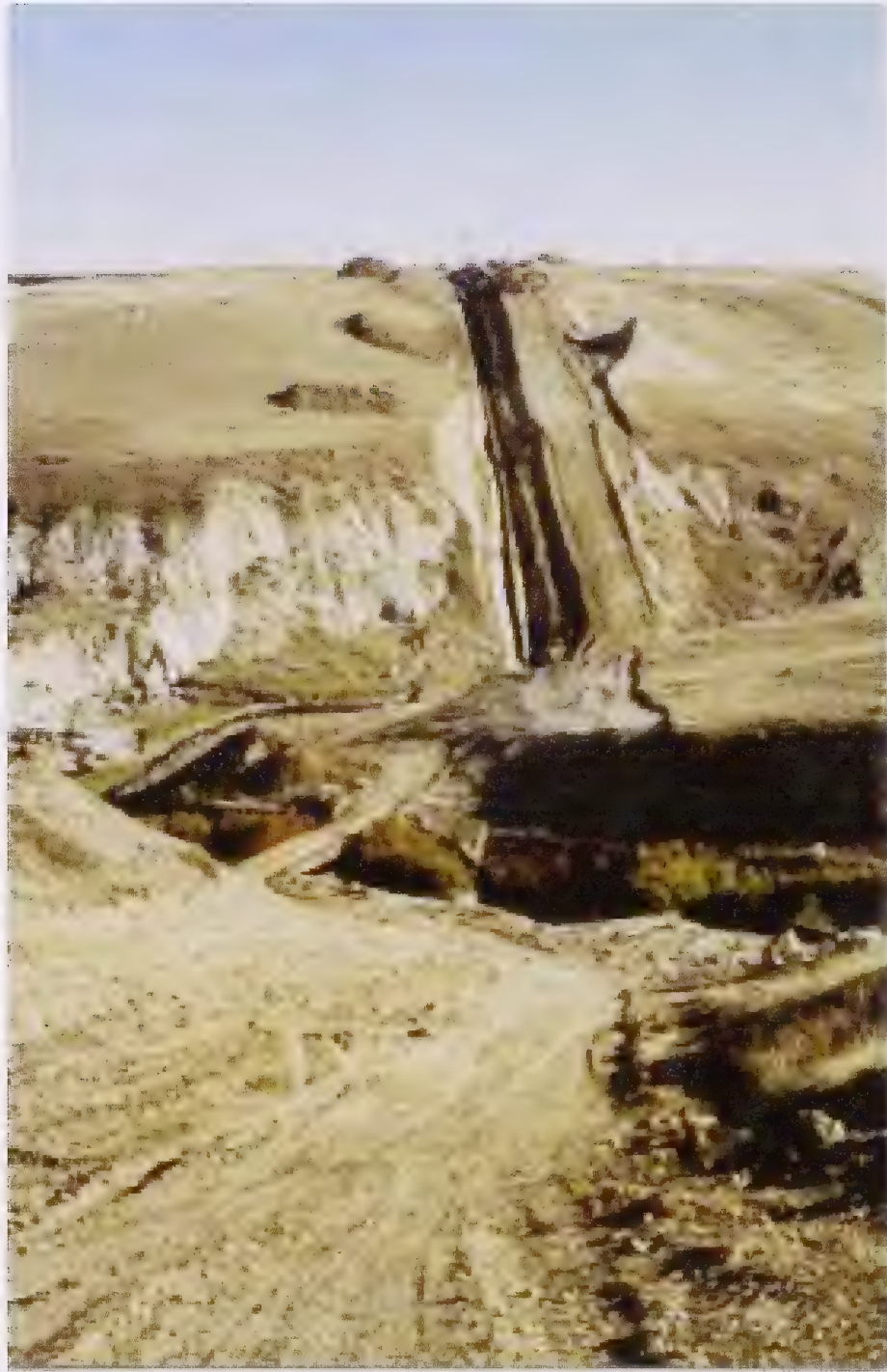
Photo 35 Grading was substantially reduced using minimal disturbance construction procedures
